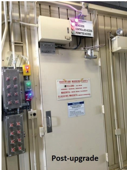
Figure 3: Sector 24 entry way.
