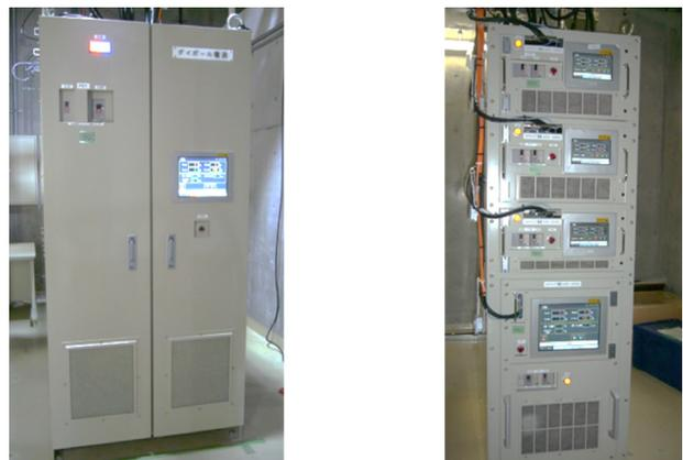
Figure 2: The pictures of a new part of power supplies for normal-conducting magnets. The left is power supply for dipole magnet and the right is four steerings installed in a rack.
