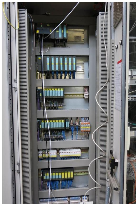
Figure 4: Main cabinet with PLC and 3 ET200S systems.
