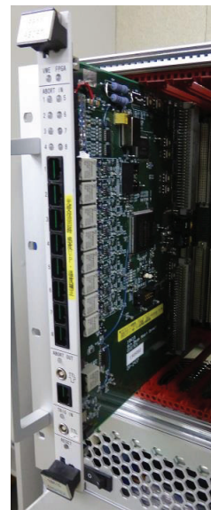
Figure 2: Picture of the VME-based 8ch beam abort optical input module (18K15).
