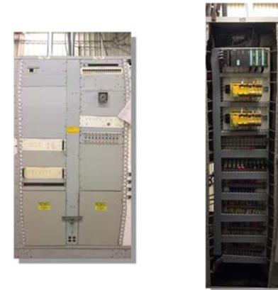
New Terminal Cabinets and approx. 4000m of copper trunking was prewired. At install, the legacy system was removed including cable plant, and the conduit was inspected and repurposed. The rack subassembly was installed in the cleared out rack and trunks terminated. New field hardware was installed and terminated at the terminal blocks.
