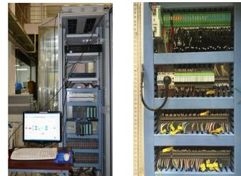
Fig. 4 Left: The ion sources control system based on PLC of Siemens S7 series 300.
